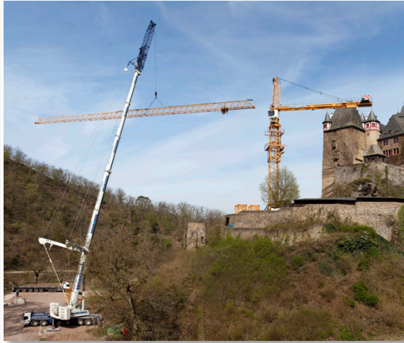
Tower crane assemblies
