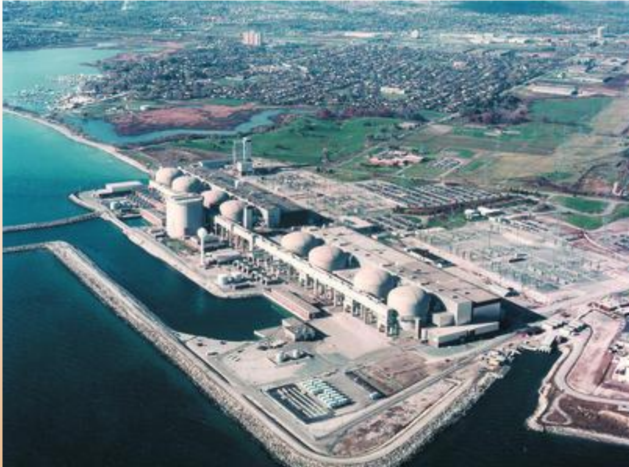
Pickering Nuclear Power Station
