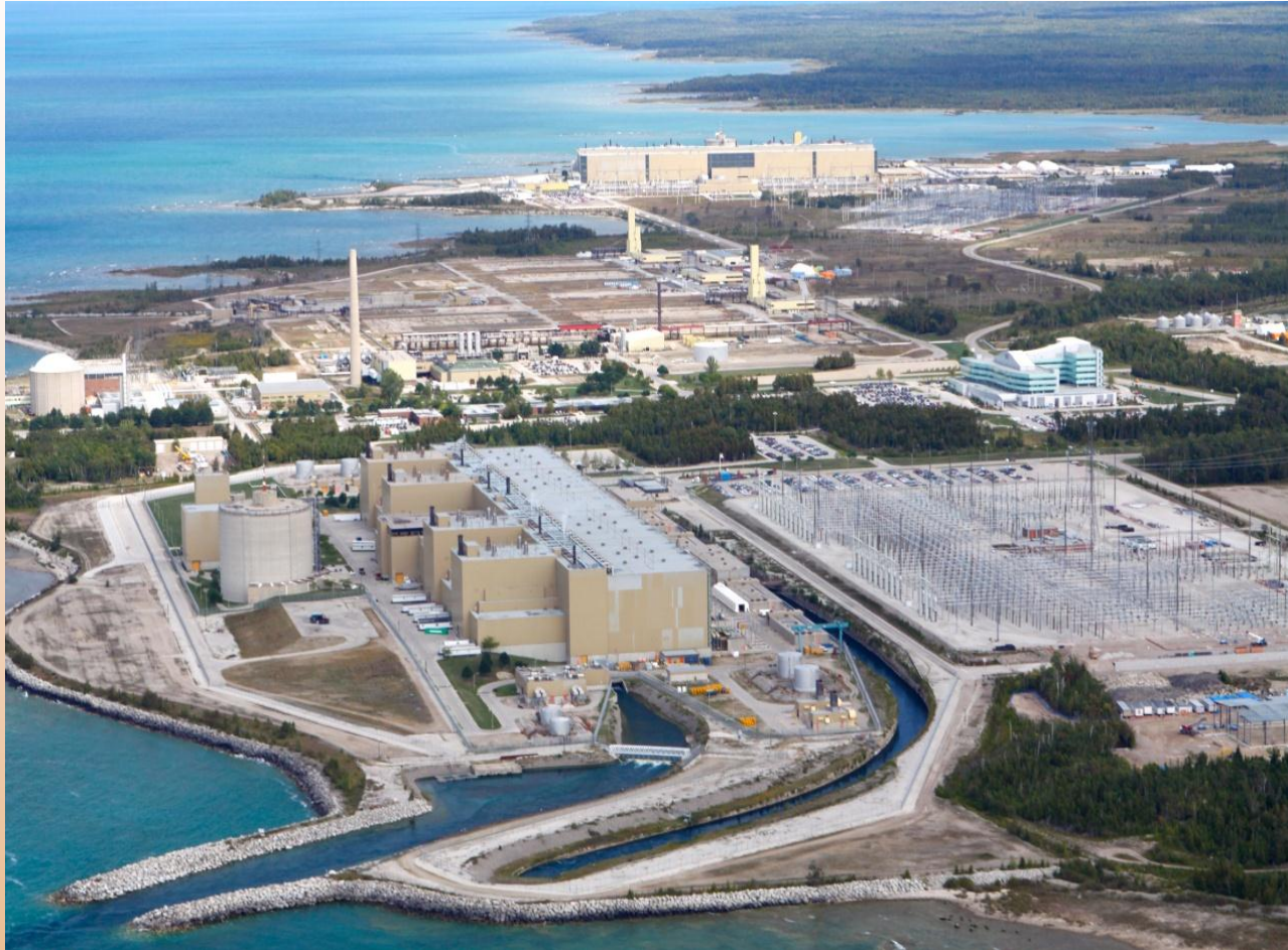
Bruce Nuclear Power Site
